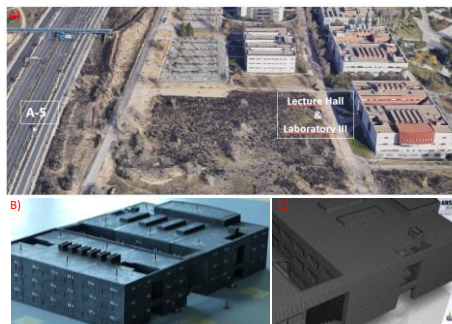
Figure 1. A) Location of the studied building, particularly exposed to pollution from the adjacent road (Google maps). B) 3D printed and C) Computational model for the realistic studied buildings.
