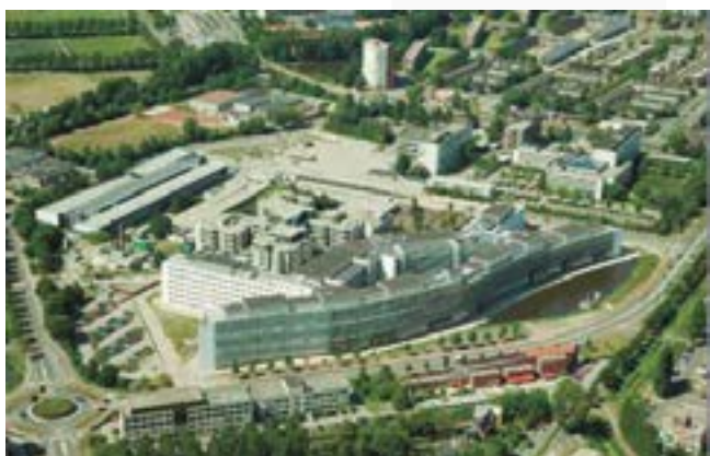
Martini Hospital, Groningen, Netherlands © Burger Grunstra consulting architects
