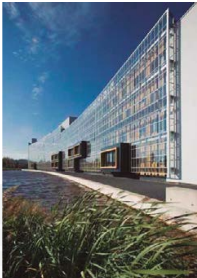
Martini Hospital, Groningen, Netherlands © Burger Grunstra consulting architects
